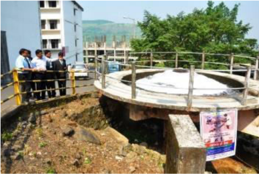
Visit to Water Treatment Plant
